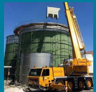
Internal settlers are substituted by ICX ® internals
