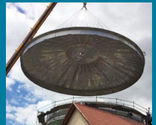
Roof of existing EGSB tank is removed
