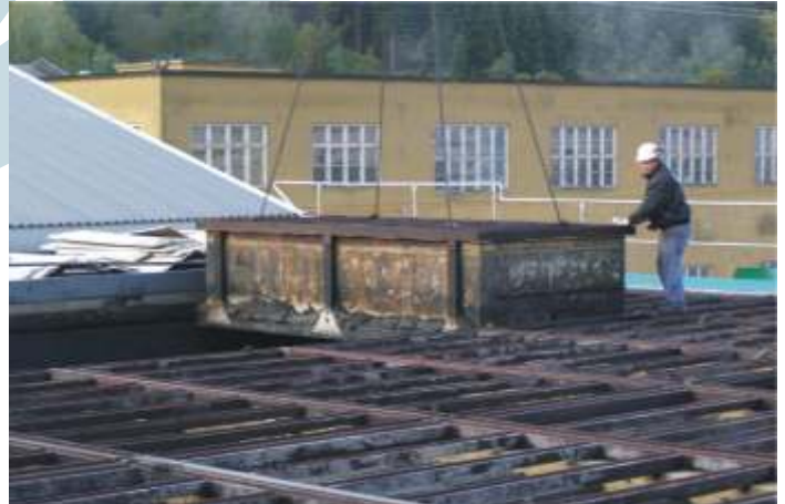
2. Removal of a settler module.
