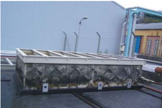
3. Putting frame in place.
