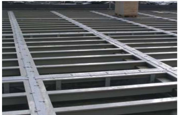
4. Even and neat surface of the retrofitted reactor.
